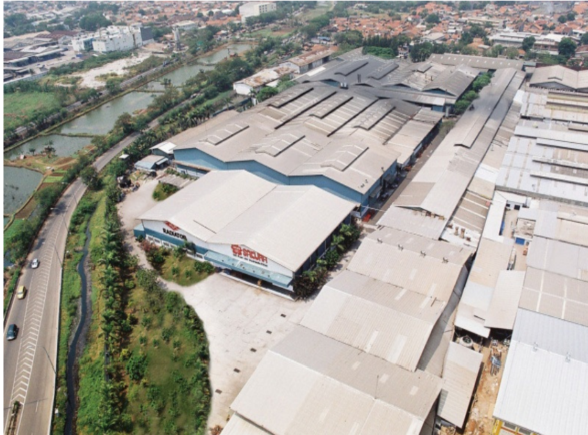
Kapuk Plant (Radiator Facilities)
